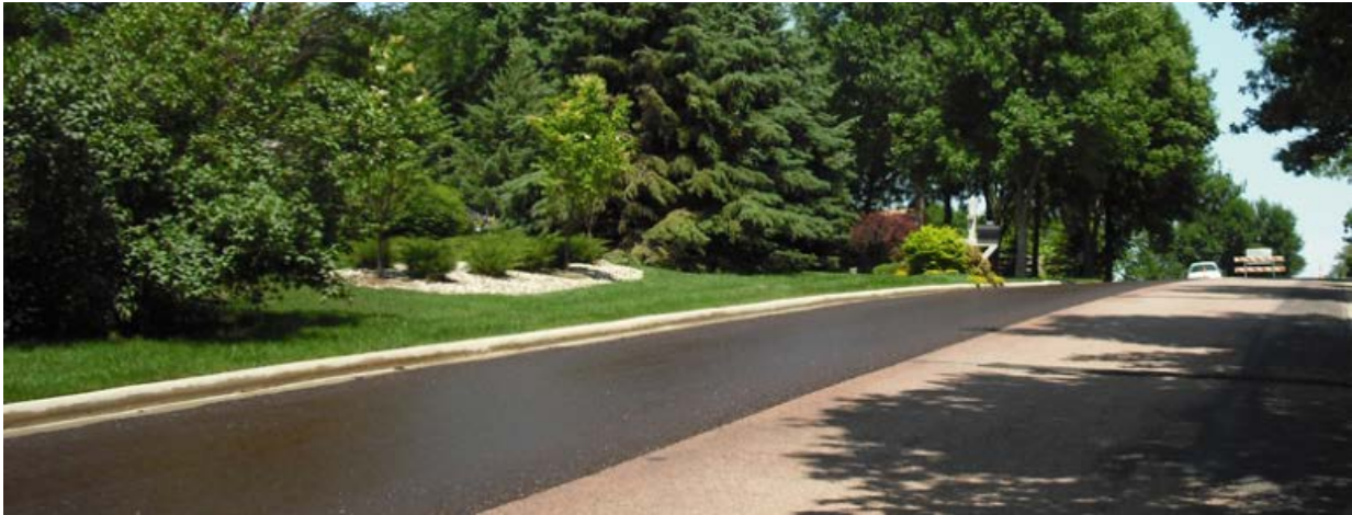
Figure 2.17: Application of Microsurfacing
