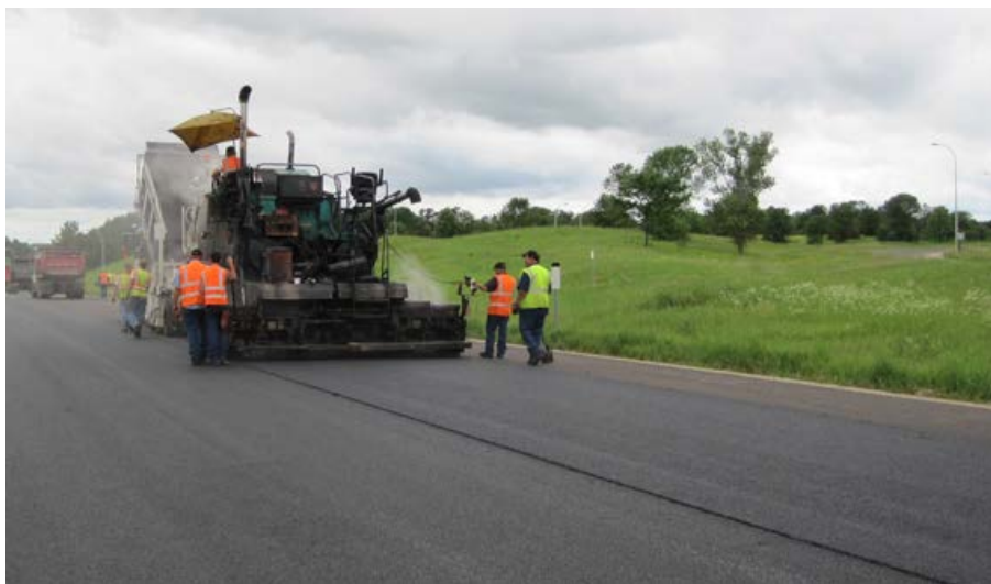
Figure 2.19: Thin Bonded Wearing Course Application (Wilde et al., 2014)
