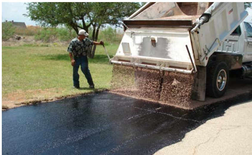
Figure 2.12: Applying a Chip Seal Layer on a Paved Road (Hafez, 2015)
